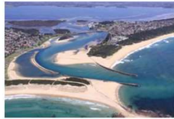
2009: trained entrance, with twin breakwaters and southern training wall fixing the entrance opening position.
